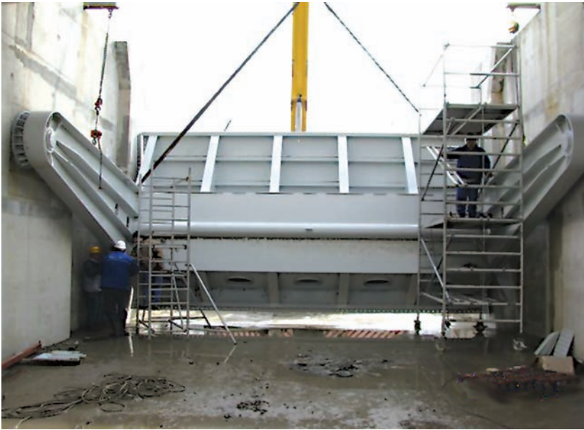
One of the segment plates of the northern structure during installation
