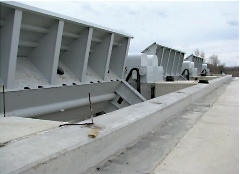
Segment plates shot from the top of the structure
