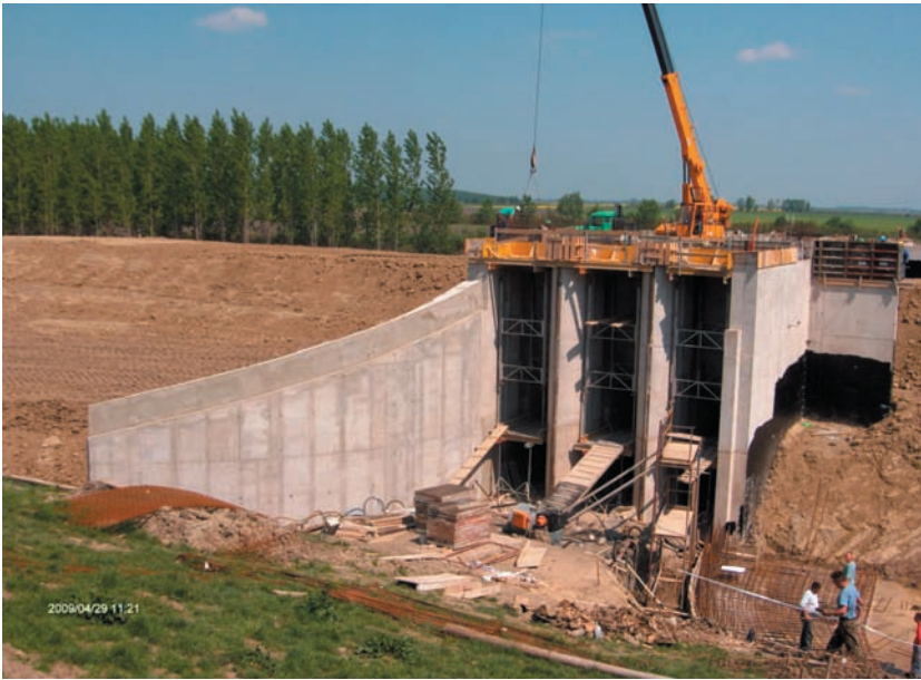
The southern structure under construction
