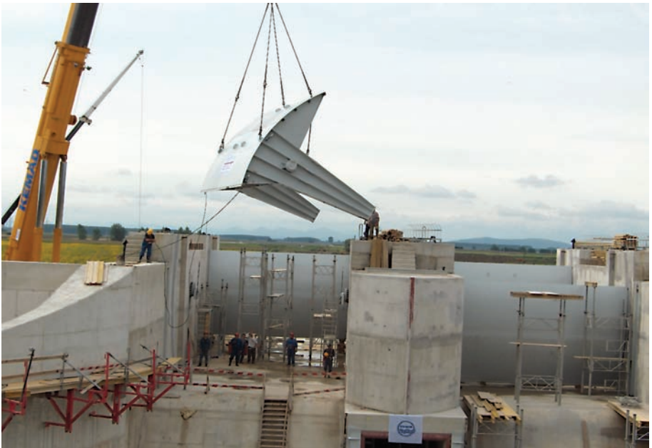
A segment plate of the inlet structure during installation
