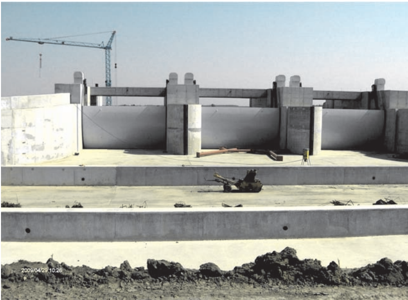
Segment plates of the northern structure from the flood plain
