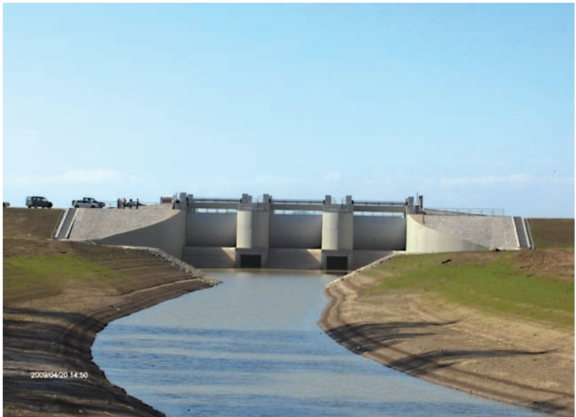
The hydraulic structure with the inlet channel, seen from the River Tisza
