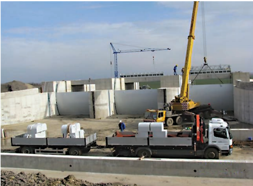
Installation of segment plates in March, 2009
