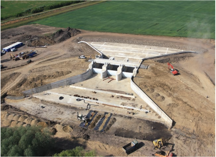
The structure under construction in May, 2009
