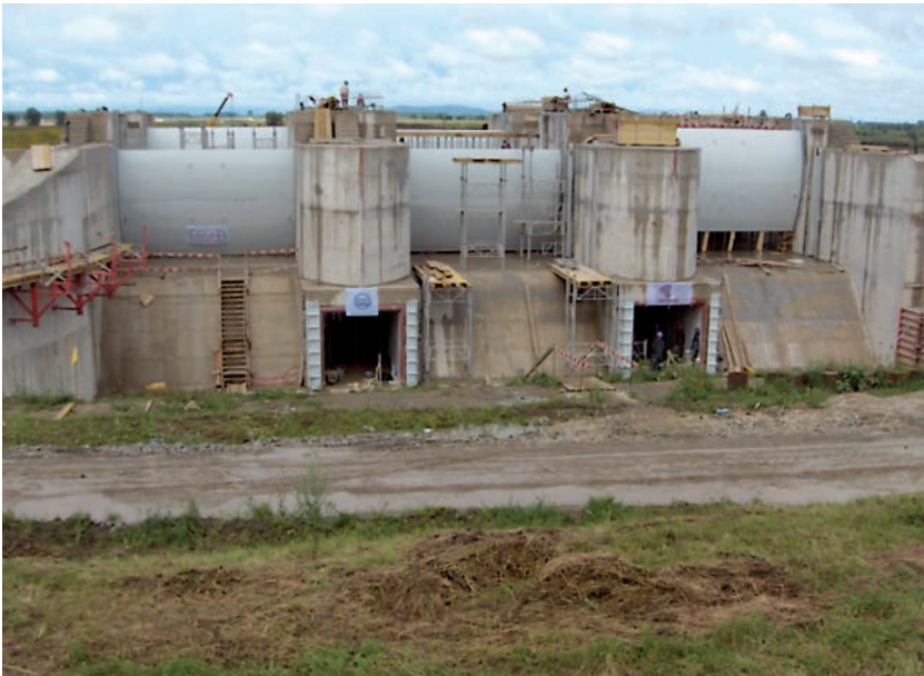
Installed segment plates in July, 2008
