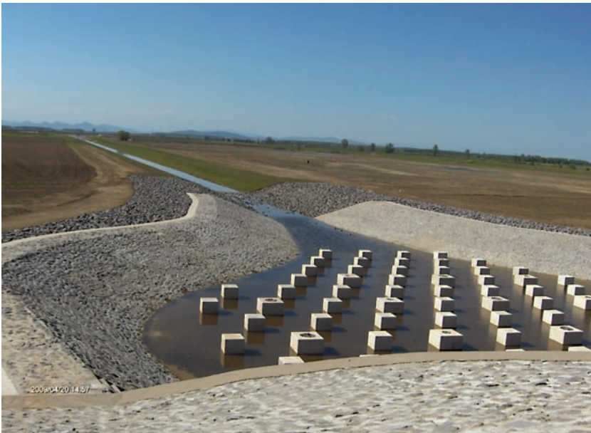
Baffle blocks in the stilling basin of the inlet structure
