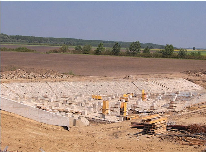
The stilling basin of the southern structure under construction
