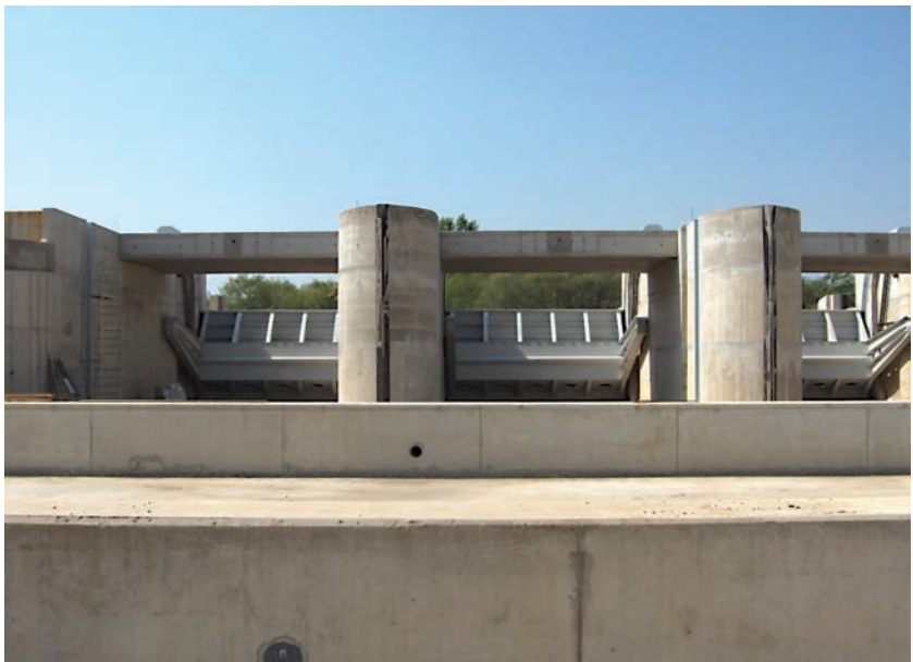
Segment plates of the northern structure from the protected side
